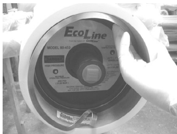
Removing the retaining ring from the groove
