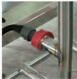
Flow Sensor Installation
