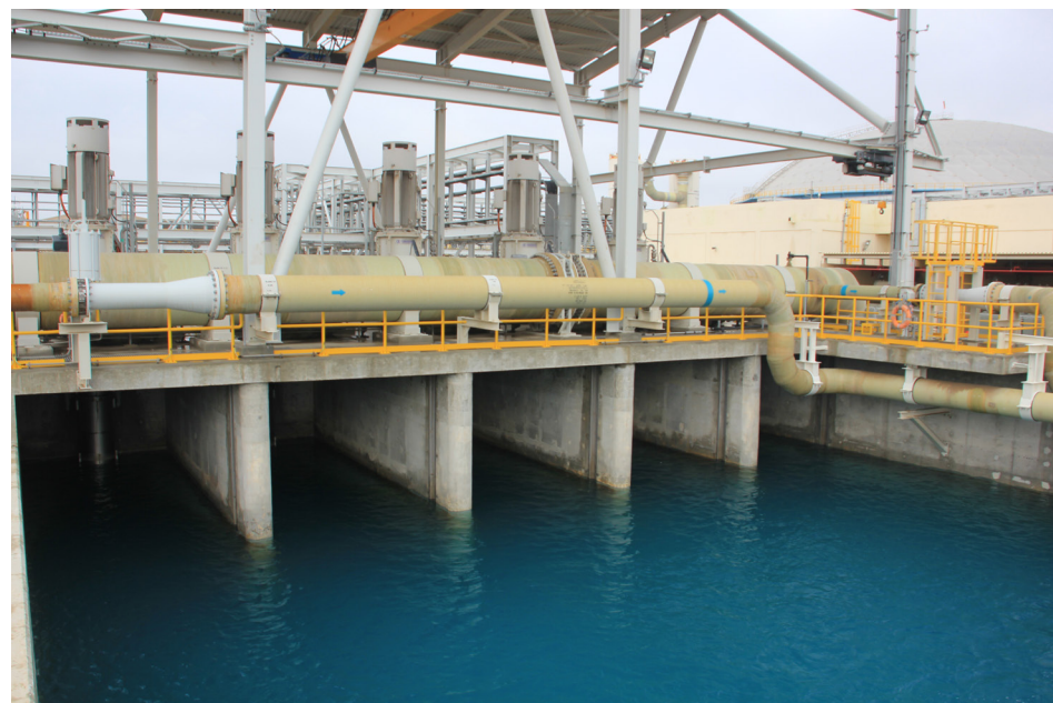
Product water storage tank for cooling tower make-up water.
